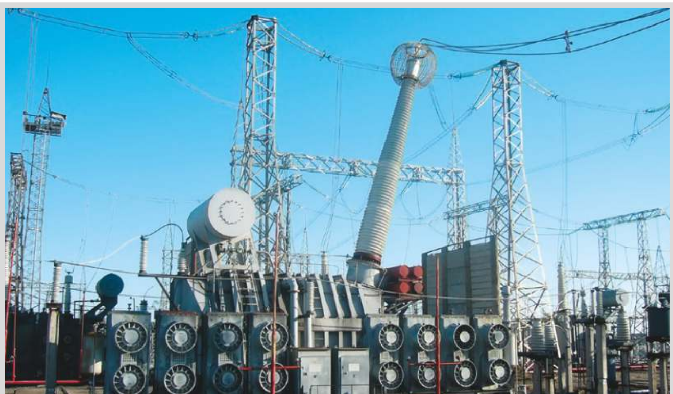
1150 kV Izolyator bushing on a 300 MVar shunt reactor. Itatskaya substation at Krasnoyarsk branch in MES Siberia of FGC UES JSC
