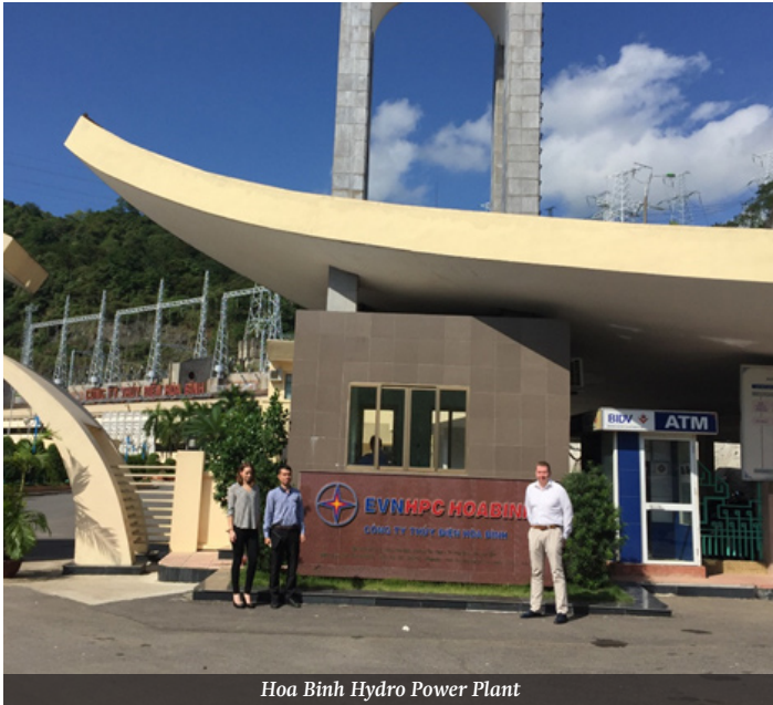
Hoa Binh Hydro Power Plant
