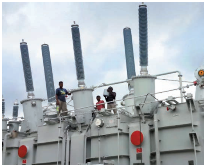
Izolyator bushings installation at SS Bamnauli in India
