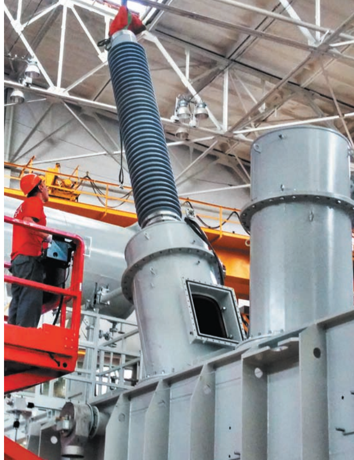
Izolyator bushings installation in a transformer by SVEL Group
