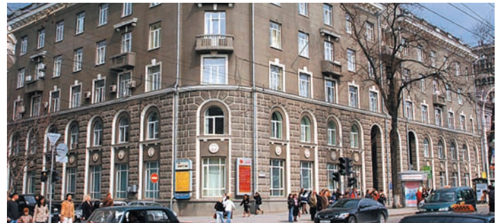
Office building Rostovenergo
