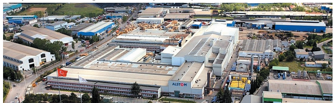
Facility in Turkey. Photo from GE website
