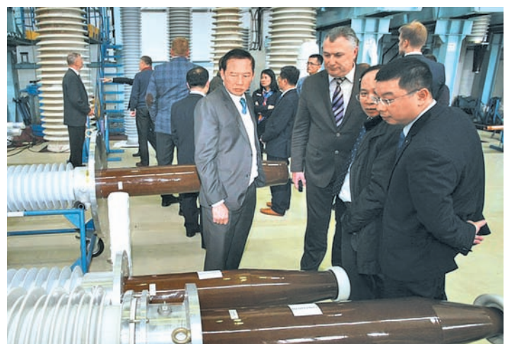
220 kV bushings assembly shop
