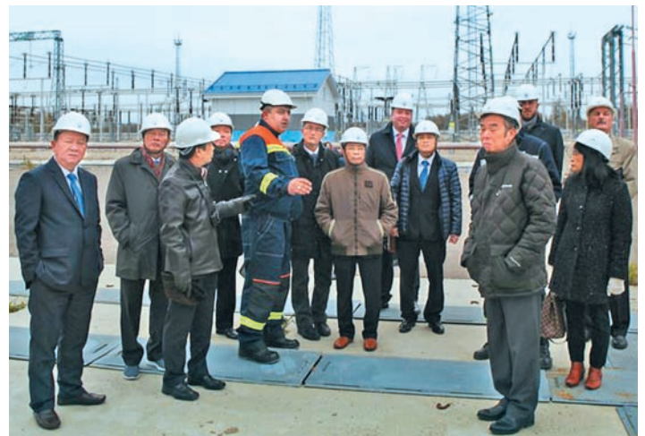
The guests are getting familiarized with modern power equipment
