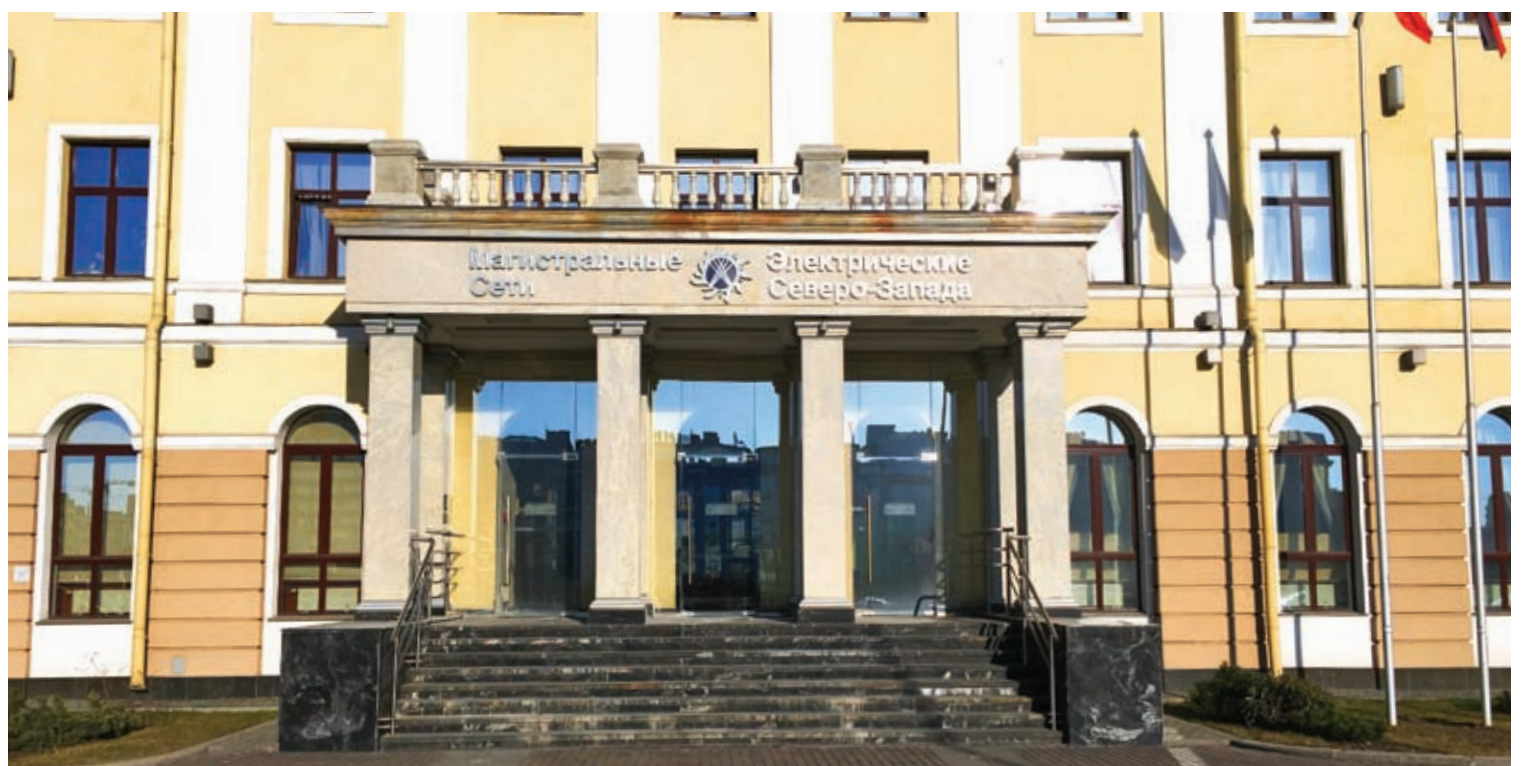
MES North West Headquarter
