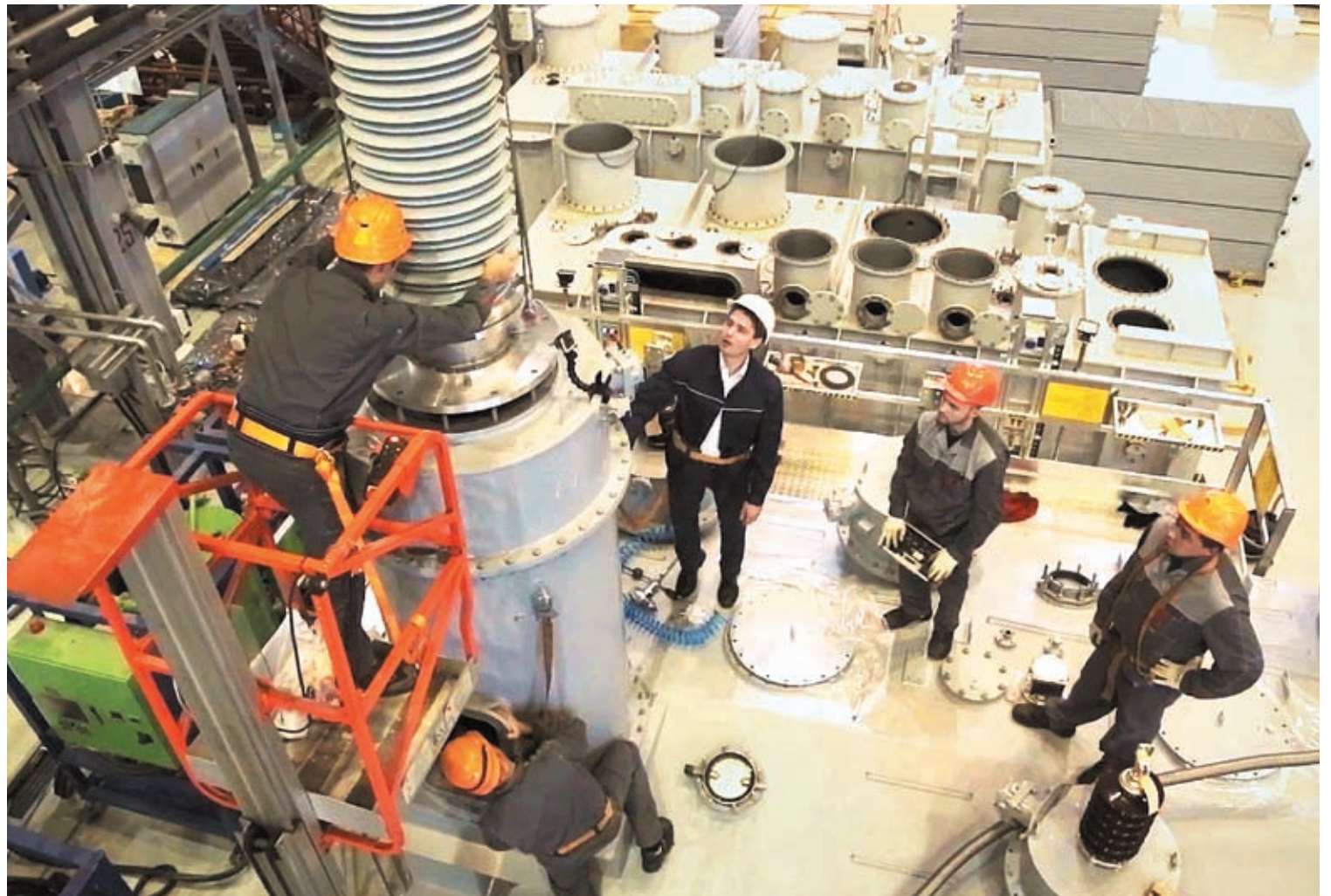
A frame from the film about Izolyator bushings installation
