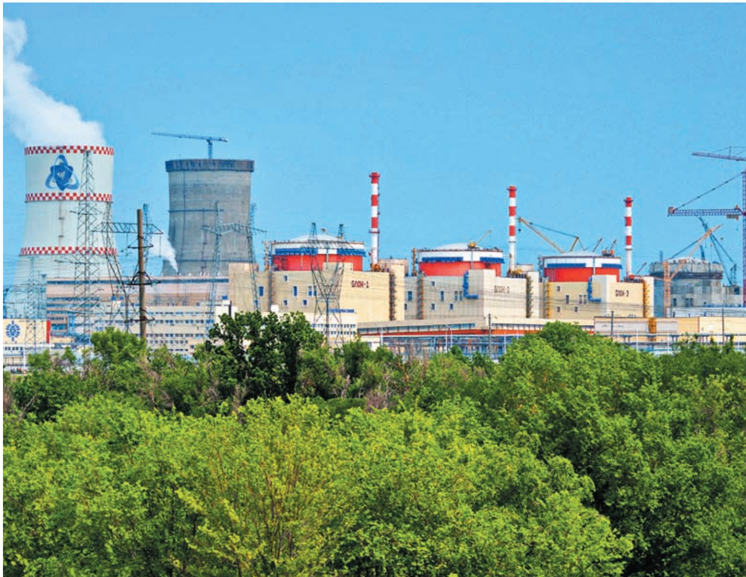
Photo from Rosenergoatom Concern's webpage
