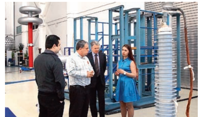
Inspection of Izolyator high-voltage bushings
