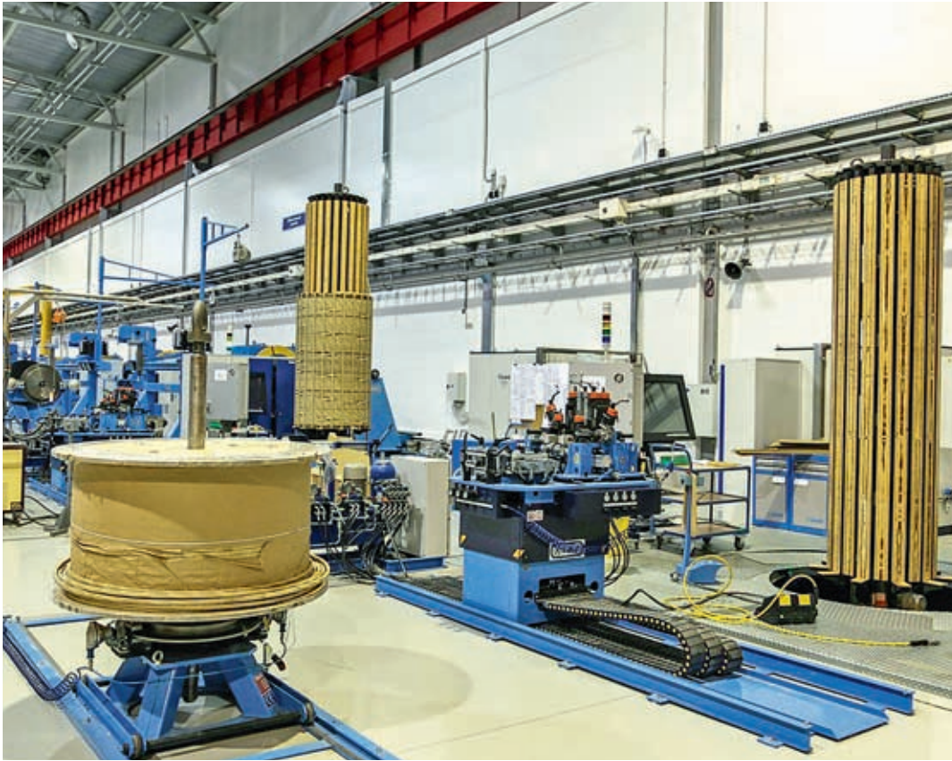
Power Machines – Toshiba. High-voltage Transformers plant (photo from Home-Made website)
