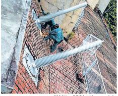
220 kV wall RIP bushings made by Izolyator delivered in 2017
