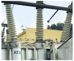
220 kV OIP transformer bushings made by Izolyator with over 25 years operation period
