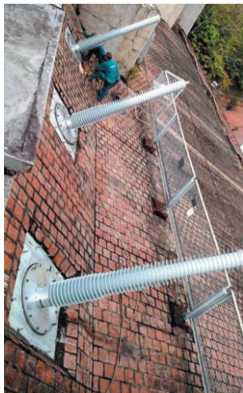
220 kV RIP bushings by Izolyator at Hoa Binh HPP
