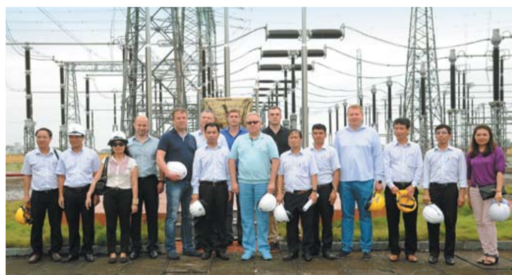
Participants of the visit to 500 kV Thuong Tin substation
