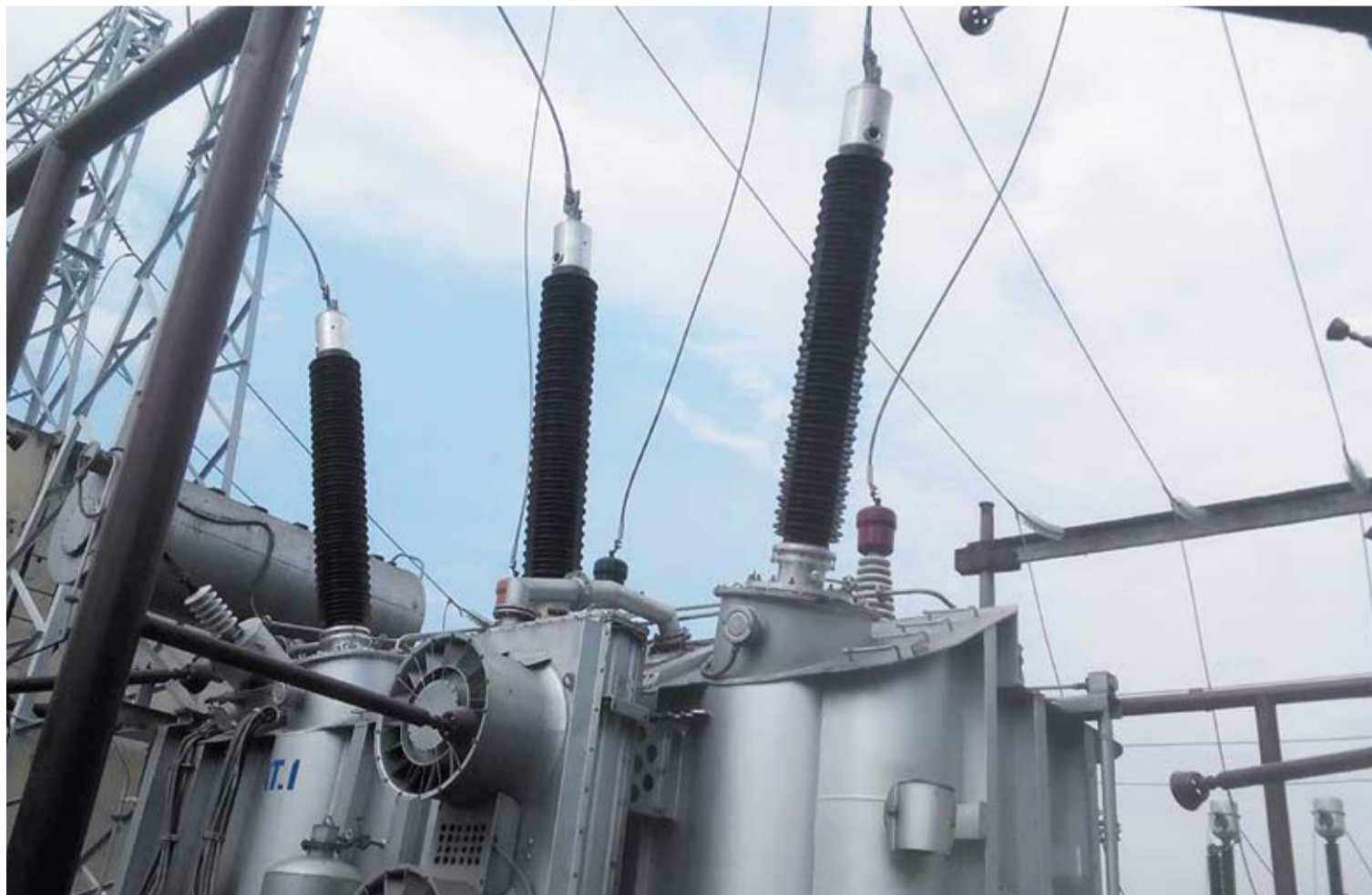
220 kV RIP bushings by Izolyator installed on a transformer at Hoa Binh HPP (Vietnam)
