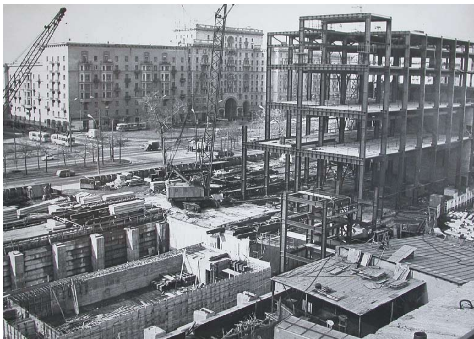
Construction of manufacturing and laboratory facility, the 1970s.
