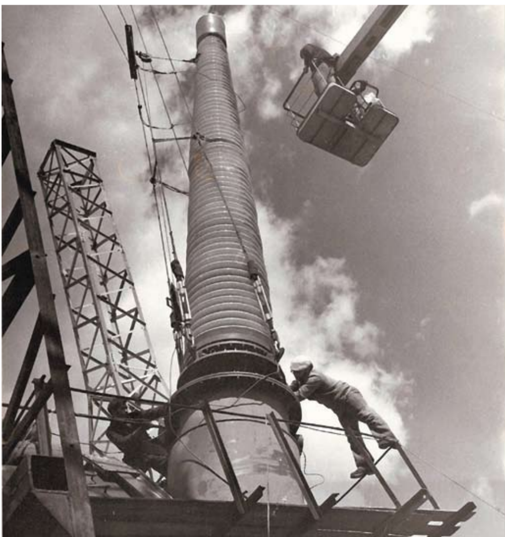
Installation of 1150 kV bushings on Ekibastuz - Kokchetav ETL in Kazakhstan
