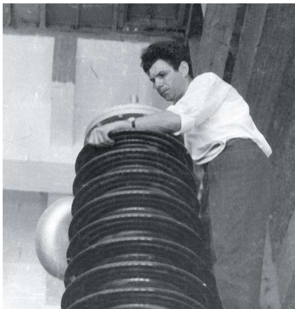
A. Barkov at the equipment installation at Aswan dam
