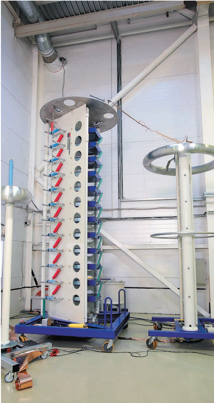
1200 kV surge impulse generator, installed at Izolyator plant's test center
