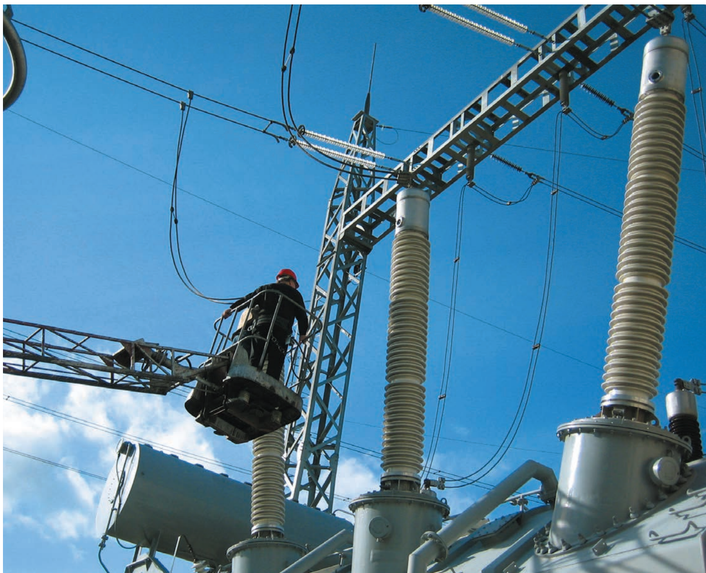
A 330 kV Izolyator bushing is getting ready for testing in Latvia
