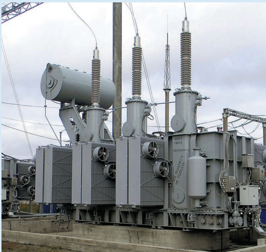
Izolyator bushings on 220 kV transformers of SS Svetlaya FGC UES (photo: FGC UES)
