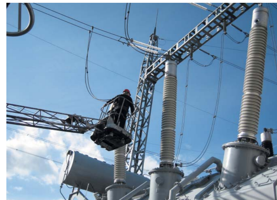
Preparation of a 330 kV bushing for testing. Jekabpils, Latvia
