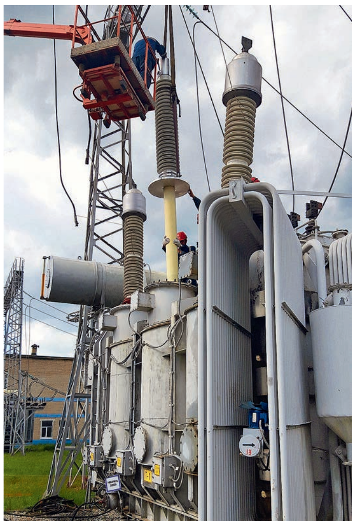
Installation of a 252 kV bushing with RIN-insulation on a 40 MVA transformer at the 220 kV Dalnyaya substation in the Vladimir region
