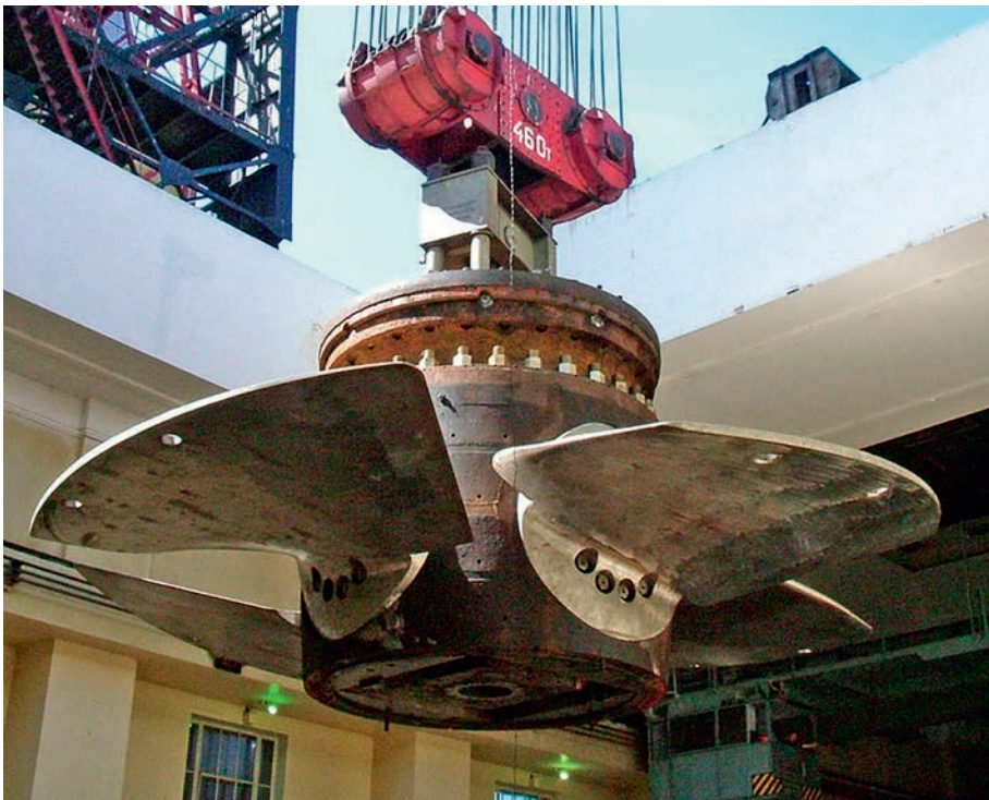
Dismantling the impeller of the Nizhny Novgorod HPP (photo: RusHydro Group)
