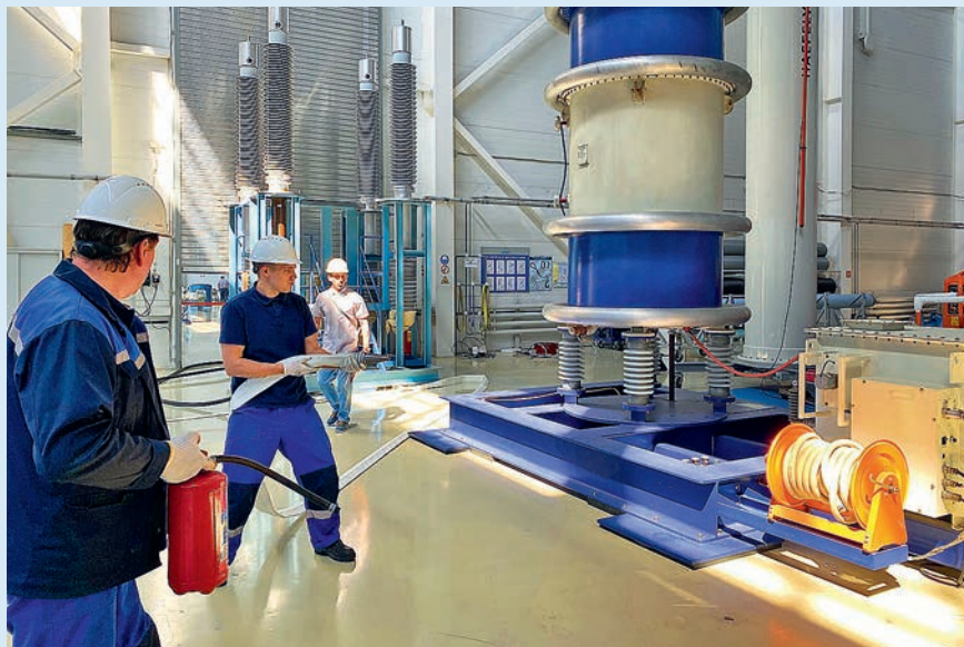
Working out skills to take actions in case of fire on electrical equipment of 220 – 1150 kV test station at Izolyator plant
