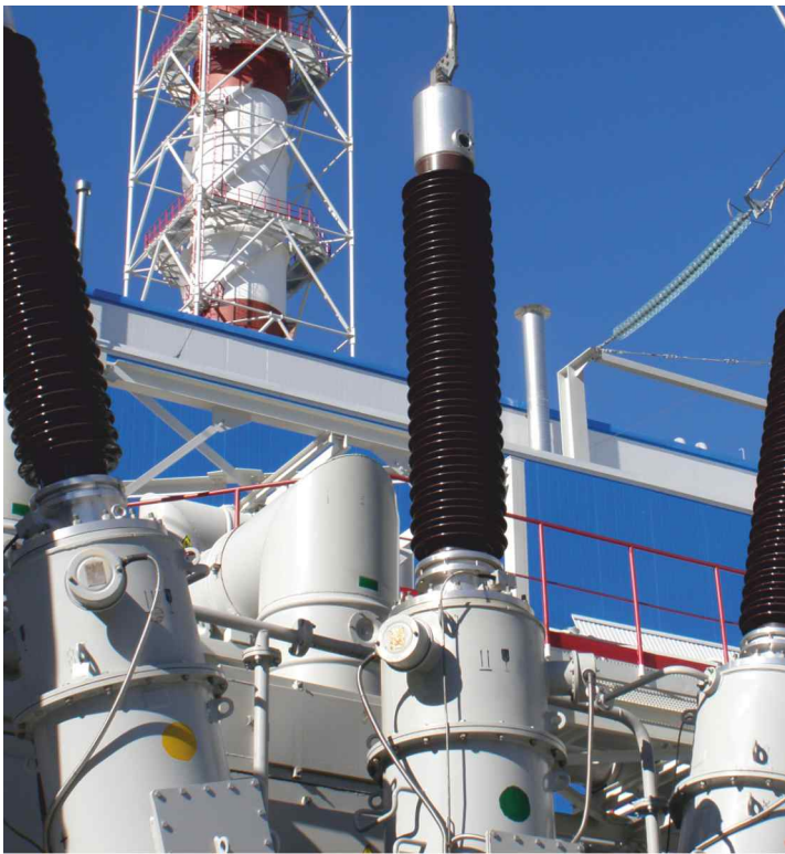
220 kV bushings in a transformer at HPP
