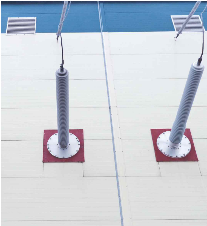
Izolyator 220 kV wall bushings in a switchgear at oil refinery
