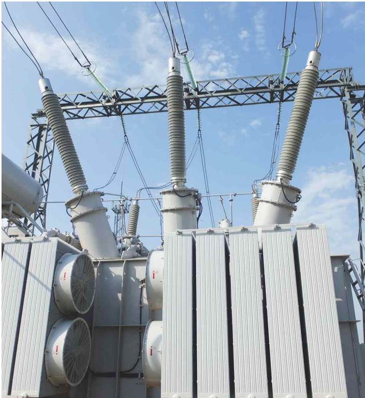
Izolyator 330 kV bushings in a Main Power Transmission Lines transformer
