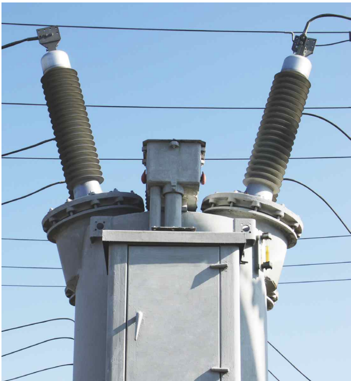
Izolyator 110 kV bushings in an oil switch of Interregional Distribution Grid Company
