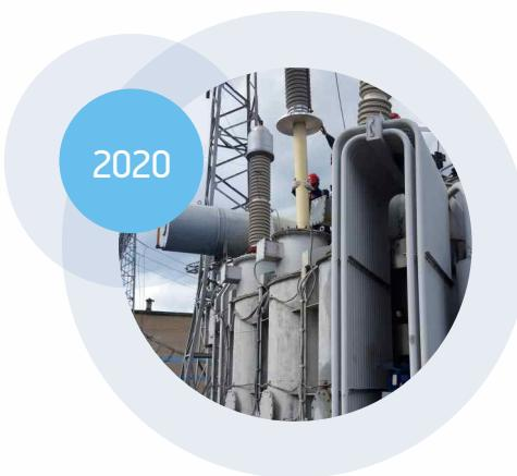
For the first time in Russia 252 kV bushing with solid internal RIN insulation was installed for pilot operation in the Vladimir region.
