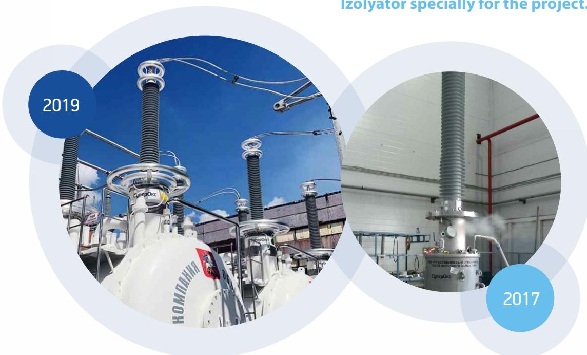
For the first time in Russia, high-voltage bushings, immersed into a cryostat with liquid nitrogen, were successfully tested at the Izolyator plant.
