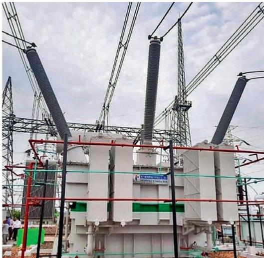
The world's first 420 kV shunt reactor with liquid ester dielectric
