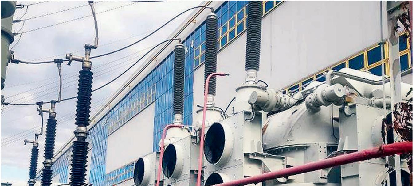
240 MVA transformer with 252 kV Izolyator bushings at Dolna Odra power plant in Poland
