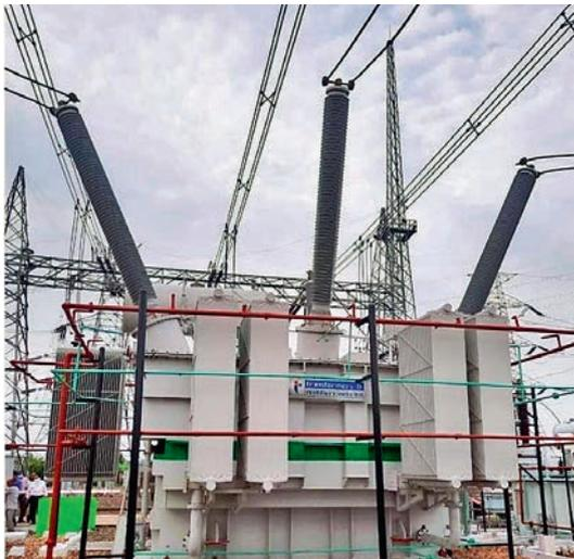
The world's first 420 kV shunt reactor with liquid ester dielectric
